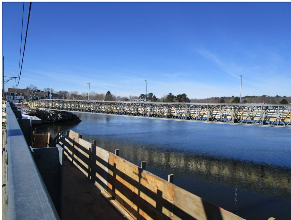
Figure 8. This close-up of the modular bridge shows the two outer truss layers, timber railing and sets of bolts that connect the panels together. Note that the surface in this photo does not represent the anticipated IPE timber deck.
