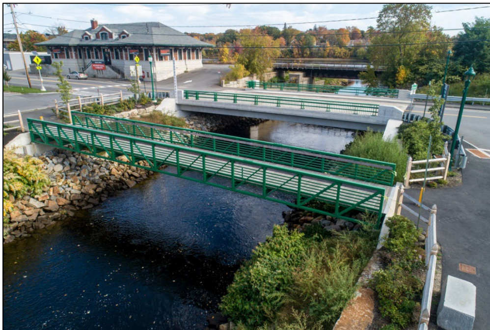
Figure 6. Prefabricated H-section truss bridge, galvanized and painted, in Gardiner, ME. This bridge was shipped in two pieces that were bolted together in a laydown area and then lifted into place as a single piece with a crane.
