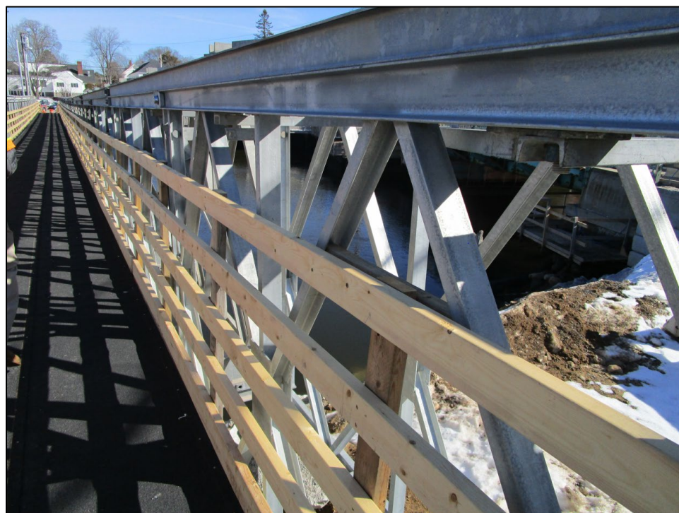
Figure 8. This close-up of the modular bridge shows the two outer truss layers, timber railing and sets of bolts that connect the panels together. Note that the surface in this photo does not represent the anticipated IPE timber deck.
